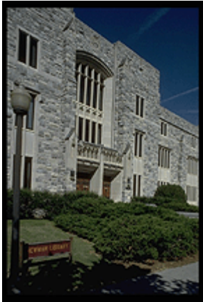
Newman Library old entrance doors. 2_76_0030 on the VT ImageBase
